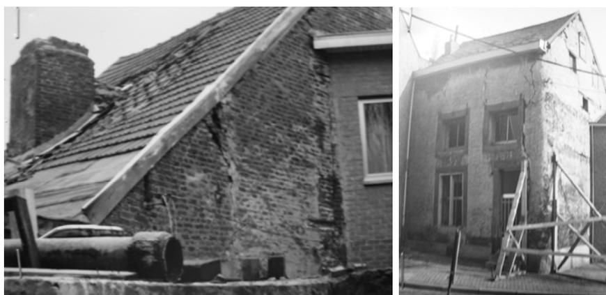
*Figure 1 - Damages on a house caused by the 1983 earthquake in Liège.*
