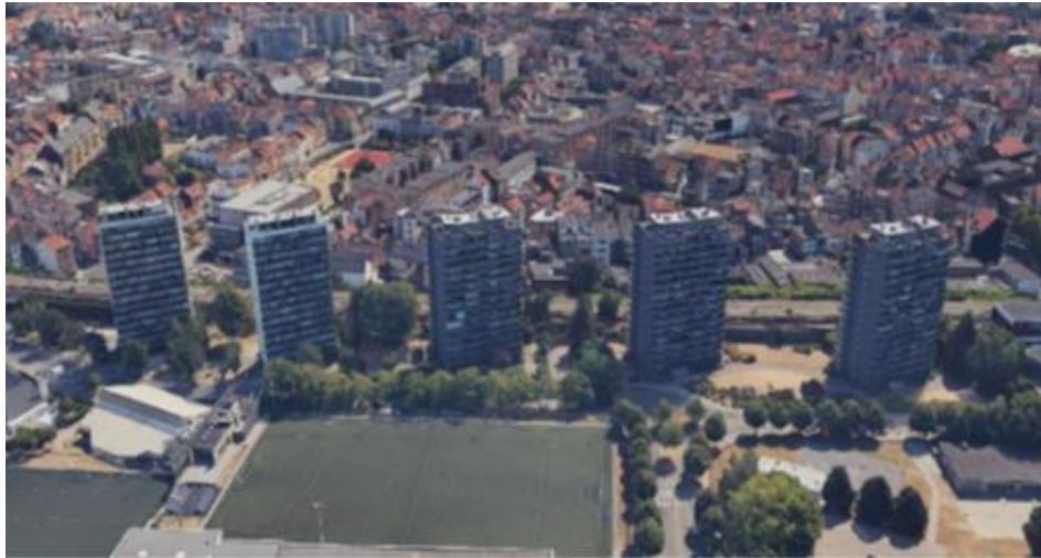
Figure 7. Ghandi apartment blocks.
