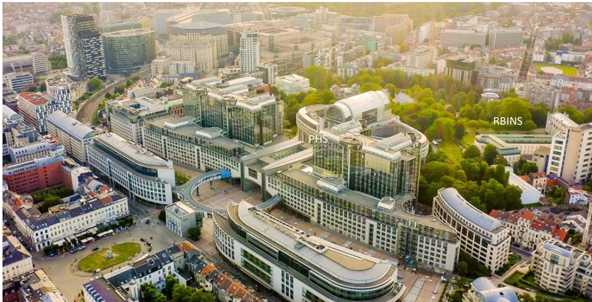
Figure 73: Aerial view of PHS and RBINS buildings
