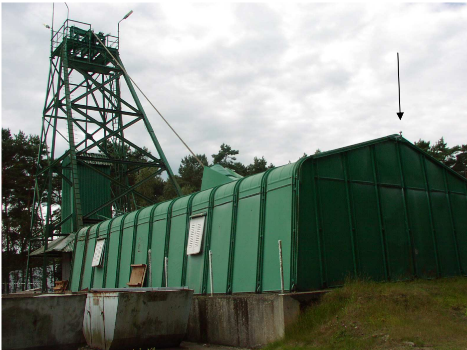
Figure 4. The GPS antenna and the old lift.
