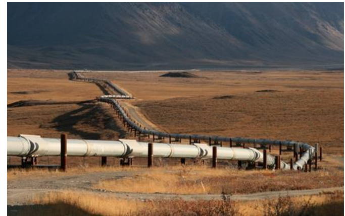
6-7 April 2000 – Pipeline corrosion, Canada
