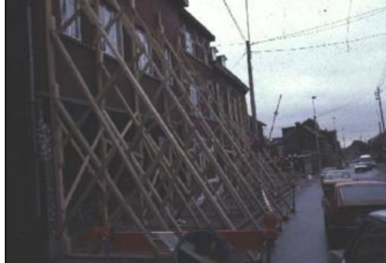
Figure 1 – Consequences of the Liège earthquake on November 8, 1983 ( M = 4.7 )
